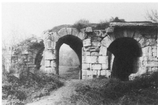
(c) Second phase vaults from east.
