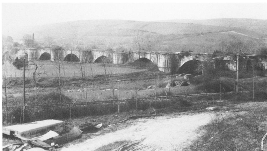
(b) South side of bridge looking west.
