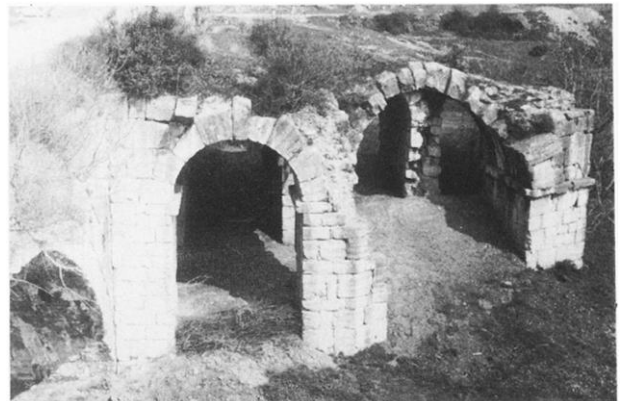
(e) First phase vaults from west.
